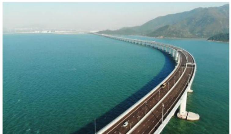
▲ Figure 1.2.1. The Hong Kong-Zhuhai-Macau bridge took over 15 years to build and cost nearly US$20 billion
