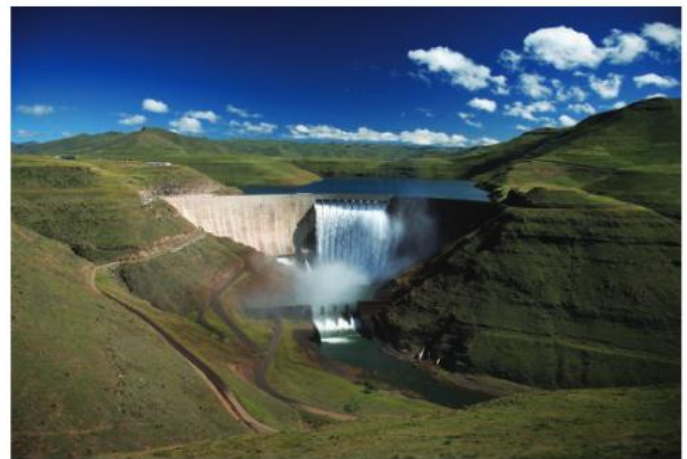
▼ Figure A.4.1. The Katse Dam in Lesotho
